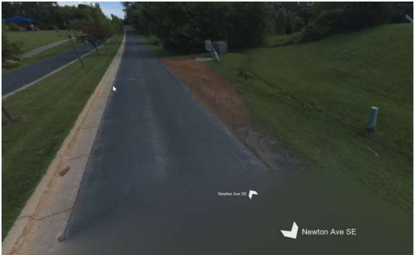
Newton Ave looking north at existing lift station.
