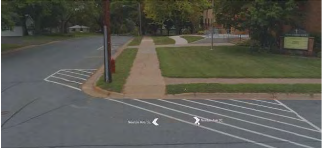
Newton Ave & Madison Street existing ADA ramp.
