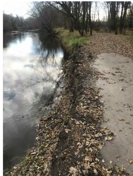
Existing Trail Looking South
